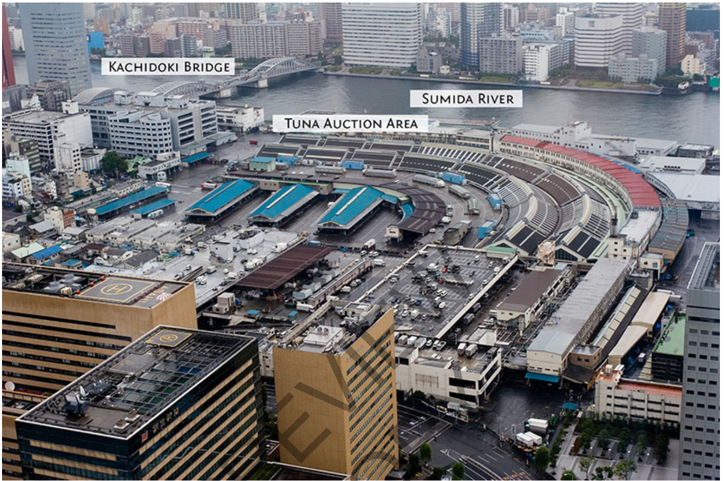
Fig. 5. Aerial view of Tsukiji market, looking southeast. Highlights added. Photo by: Ovc.
