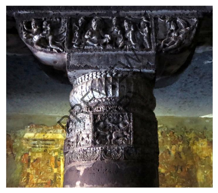
Fig. 16. Columns with compressed cushion capitals and elaborate brackets, Cave 1, Ajanta.
